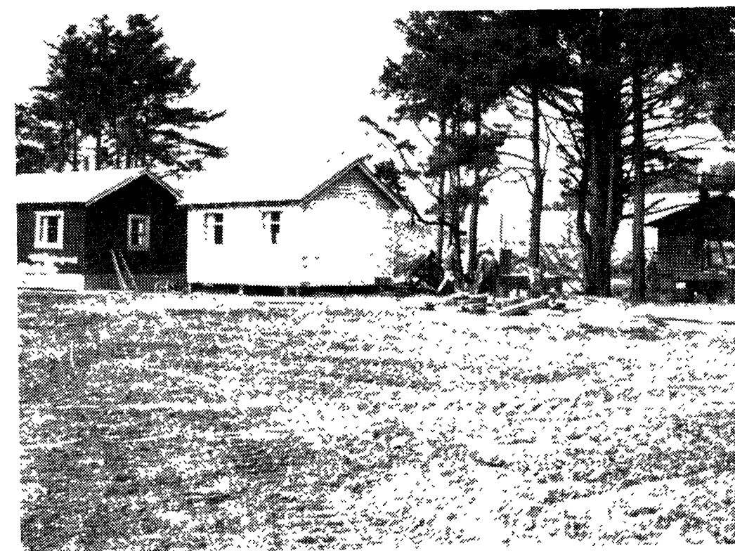
COTTAGE PREPARED FOR RELOCATION
